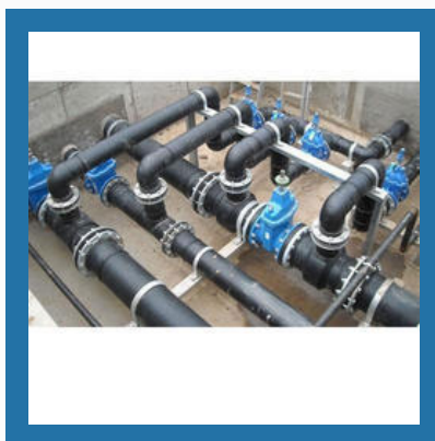
Pipe Line Service
