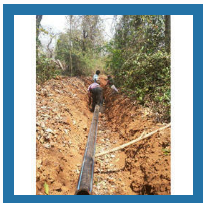
Pipe Line Installation Service
